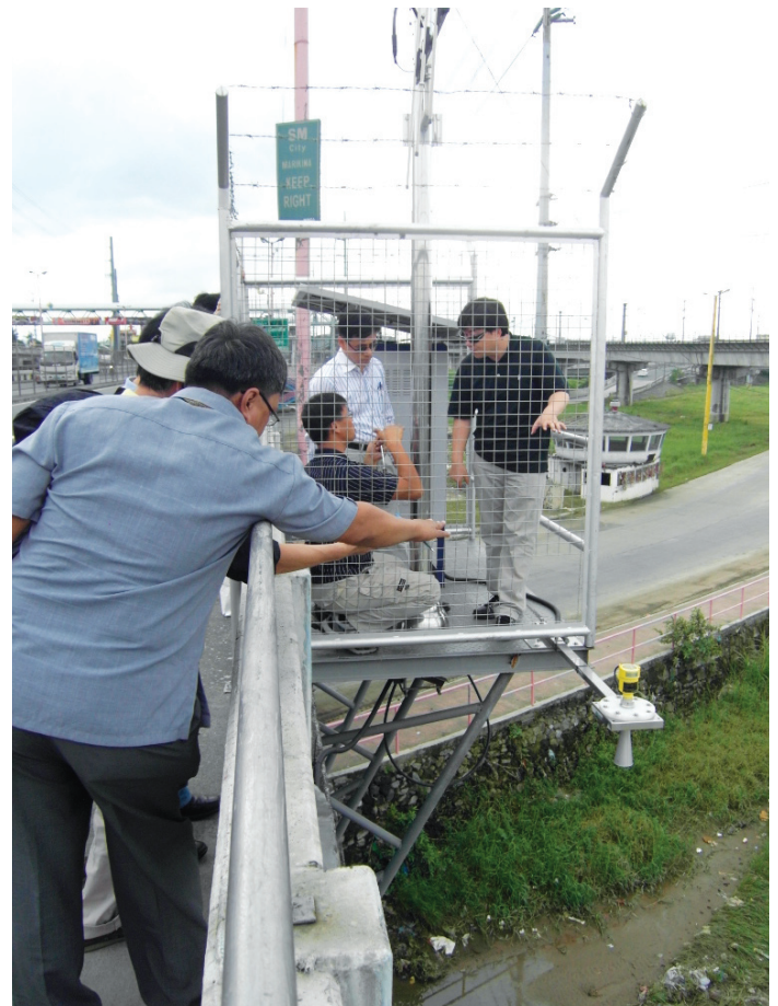
> AWS equipment installation
