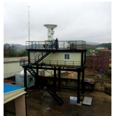
(b) installation of radar
